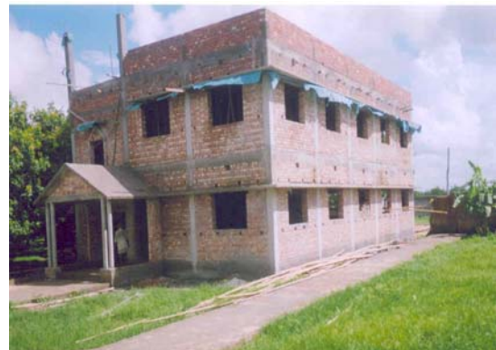
Teresa cottage under construction
